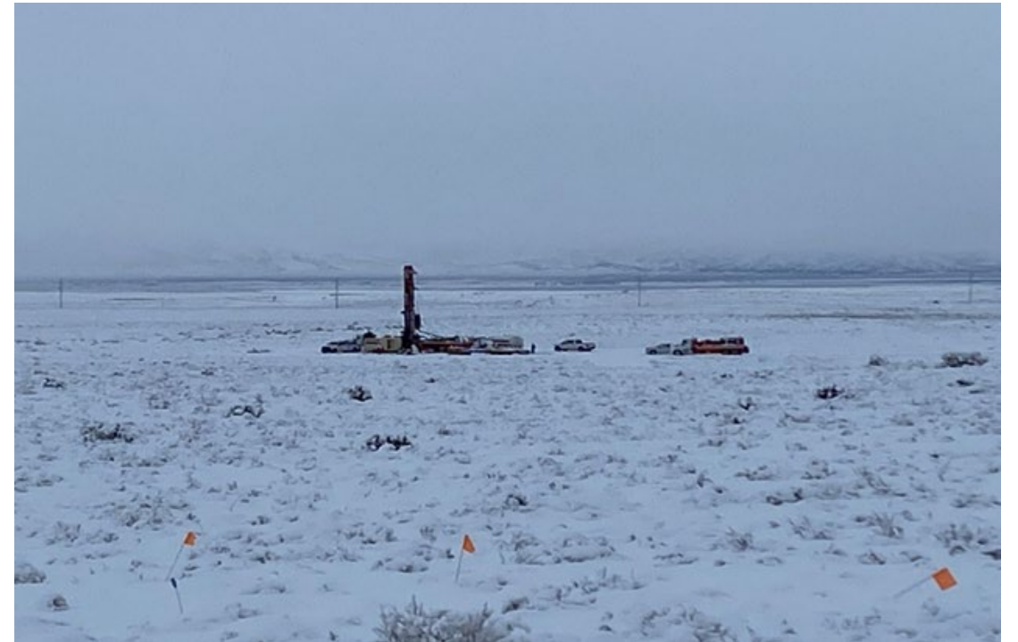
Shift 7: Well Drilling
