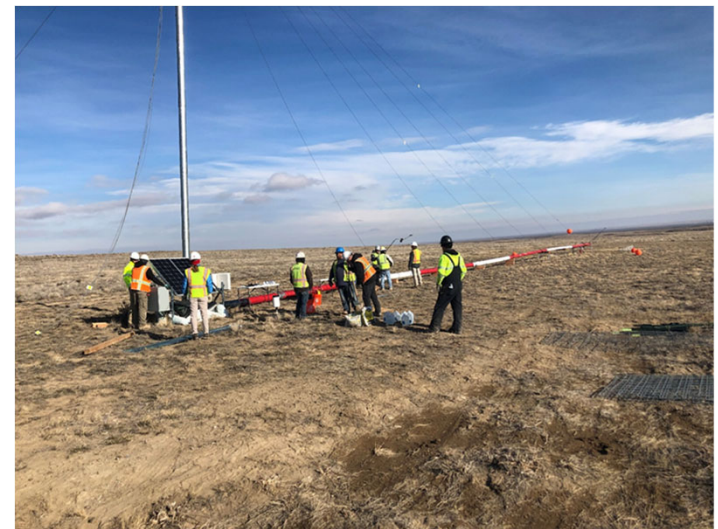
Met Tower Lowered Instrument Installation & Calibration
