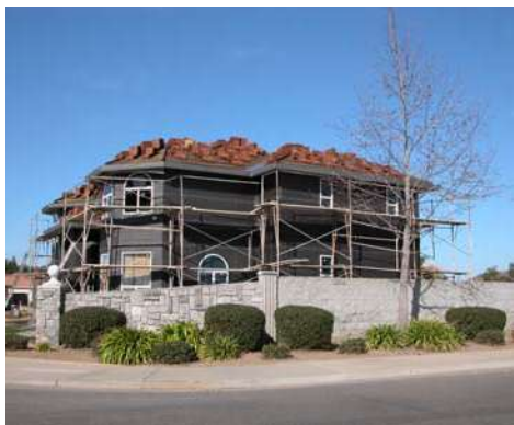
Several new residential projects were under construction in 2002.
