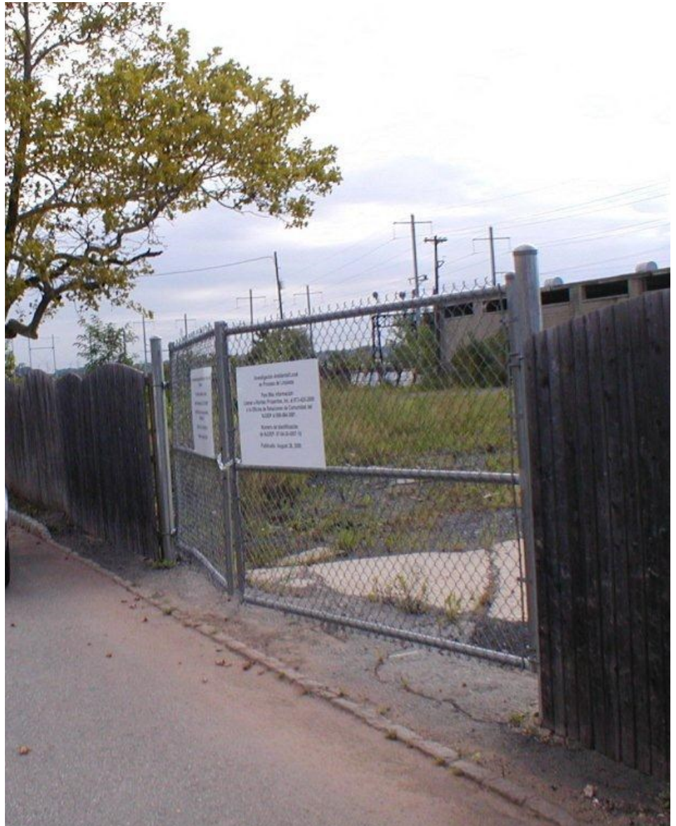
Fig. 1.3: Gates into site near center of property along 2 nd Street
