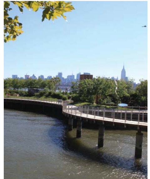
Fig. 5.10: Pier C, Hoboken, NJ
