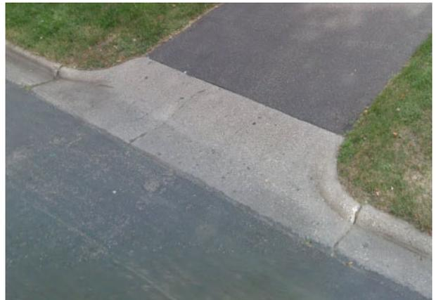
*Figure 2. Aprons like this will be replaced with asphalt behind the curb*
